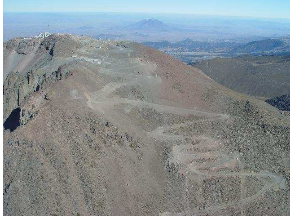
Figure 2.13: The LMT access road to the Sierra Negra summit. White boxes at the access points to the underground electric line are noticeable.
