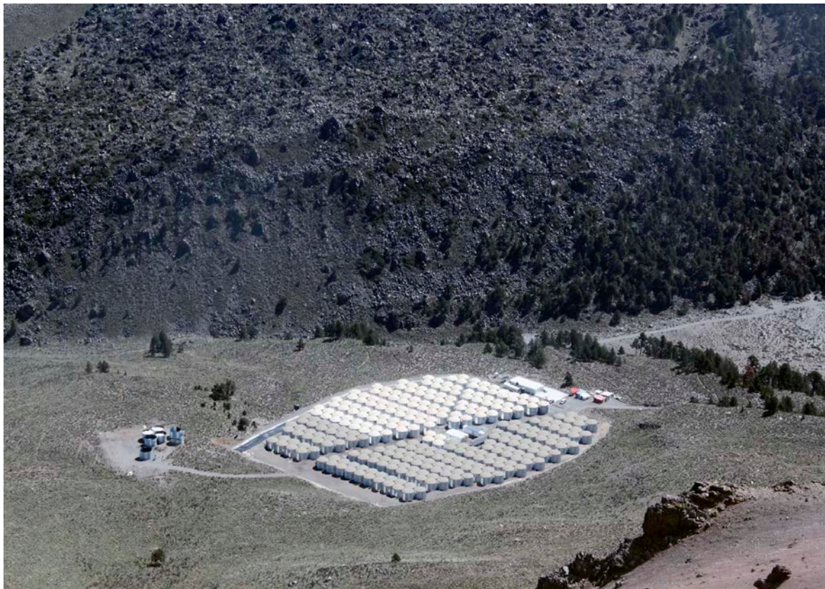
Figure 4. A photograph of the HAWC Observatory taken in August 2013 from the summit of Sierra Negra. The image has been altered to show HAWC as it will appear when construction is complete in 2014. The 111 Cherenkov detectors currently installed (100 Cherenkov detectors in operation) are colored white and located in the upper right quadrant of the array.
